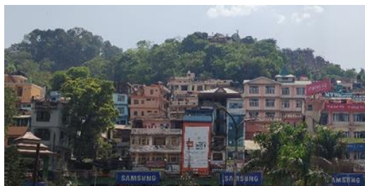
Fig. 11: Multi Story RCC Buildings near Indira Market
