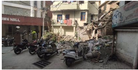
Fig. 7: Demolished Traditional Chowki House Source: Author
