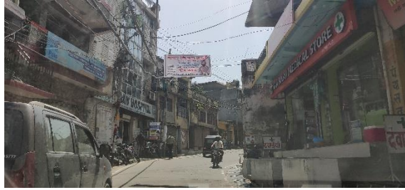
Fig. 15: Inappropriate ratio of road width and Building
