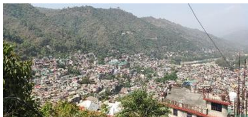
Fig. 12: Haphazard Development in Mandi town
