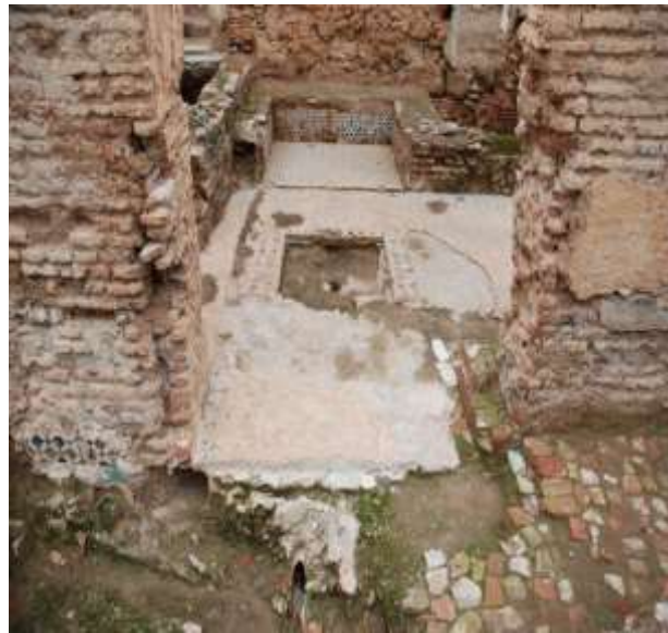
Fig. 6: The condition of the palace before the operation in 2009.
