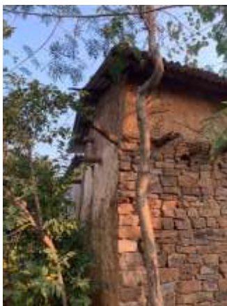
Fig. 8: Backside of a residence with exposed stone masonry Source: author
