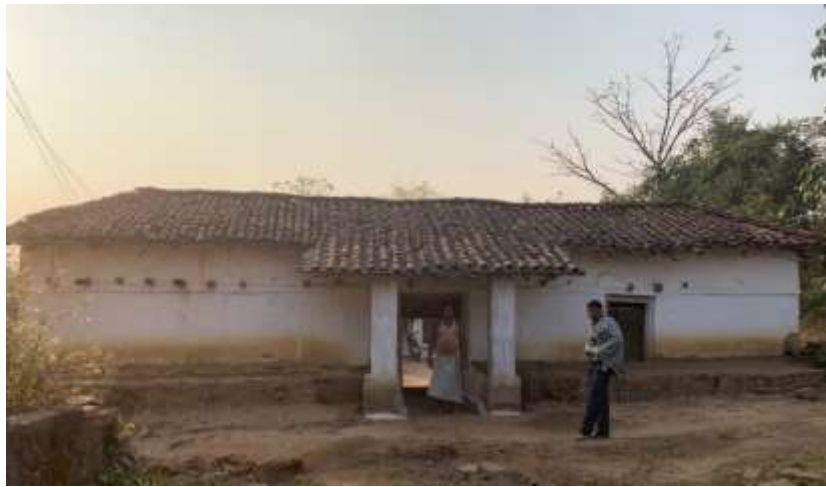
Fig. 3: Front facade of a house at Khudargad
