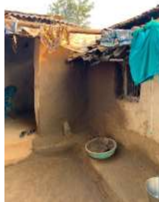
Fig. 9: Mud slurry being applied on the walls Source: author
