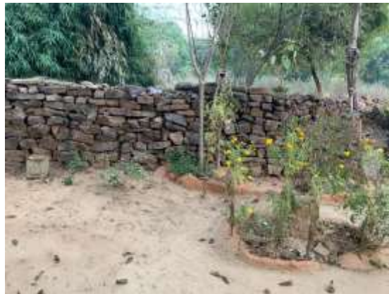
Fig. 7: Boundary wall made of stone Source: author
