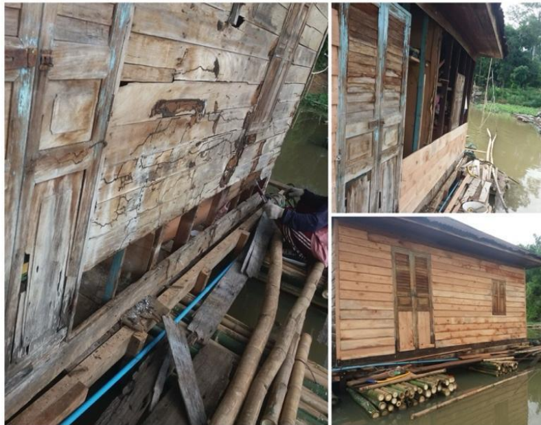
Fig. 14: Repair of walls of wooden structures Source: Author
