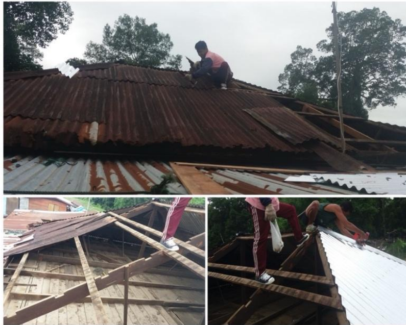
Fig. 15: Repair of the roof of a wooden structure Source: Author
