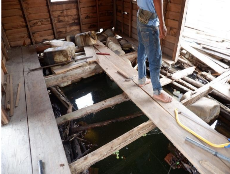
Fig. 13: Repair of wooden floors Source: Author
