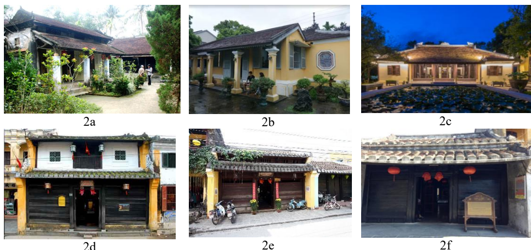
Fig. 2: Representative vernacular dwellings selected for the case studies in Central Vietnam: (2a–2c) Nha Ruong in Hue – Kim Long, Phu Hiep, and Huong; (2d–2f) Ancient houses in Hoi An – No. 33 Nguyen Thai Hoc Street, No. 62 Bach Dang Street, and No. 77 Tran Phu Street.
