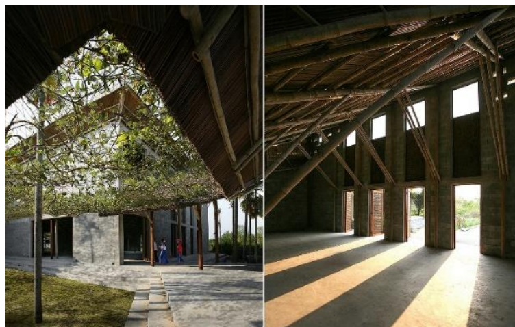
Fig. 17: Cam Thanh Community House - bamboo & non-fired brick hybrid. Source: Hao, 2013
