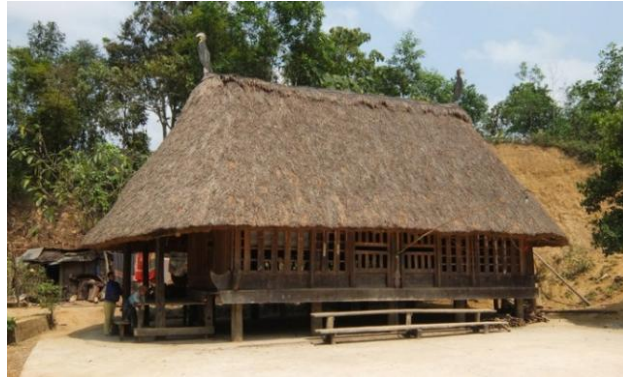
Fig. 1: Guol house in Quảng Nam province Source: Tung, et al., 2025
