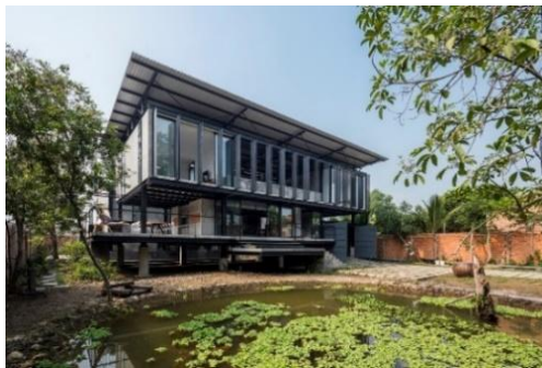
Fig. 10: Hoang Tuong House and Studio - Elevated floor Source: González, 2018
