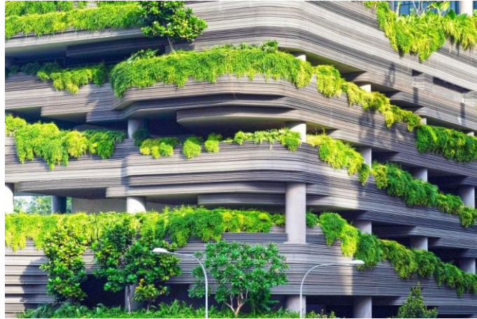
Fig 7: Transitional spaces form sky gardens that allow wind to enter and circulate throughout the building.
