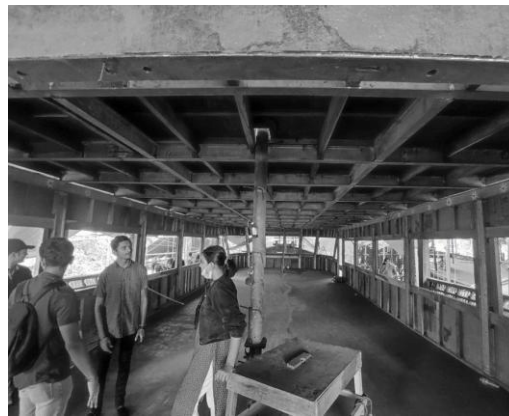
Fig. 10: Structural system of metal and wood for the upper-level cabin
