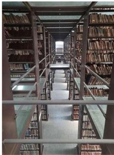
Fig. 8.2: 1.2-meter-wide passage and 2-inch-thick Belgium glass measuring 90 cm x 75 cm. Source: Author, 2024.
