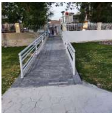
Fig. 13: Secondary entrance with ramp without tactile surface or construct warning strip Source: Author
