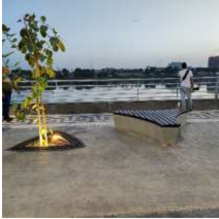
Fig. 16: Grating covering the plant with openings more than 13 mm Source: Author
