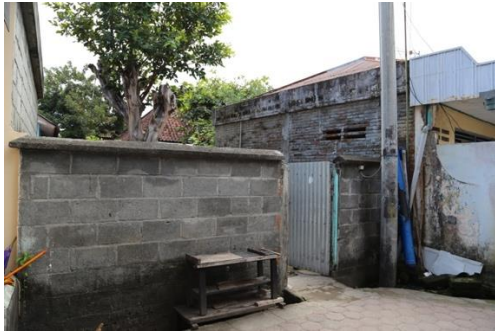
Fig. 2: Main entrance gate Source: Authors, 2018
