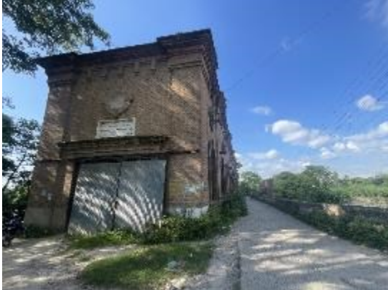
Fig. 23: Bahadarabad power house built in 1930, Bahadarabad.
