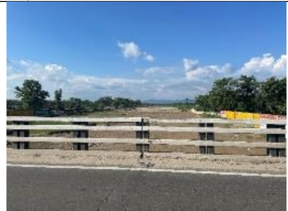
Fig. 22: Canal passing below Rutmoo river in Begampur. Source: Authors, 2024
