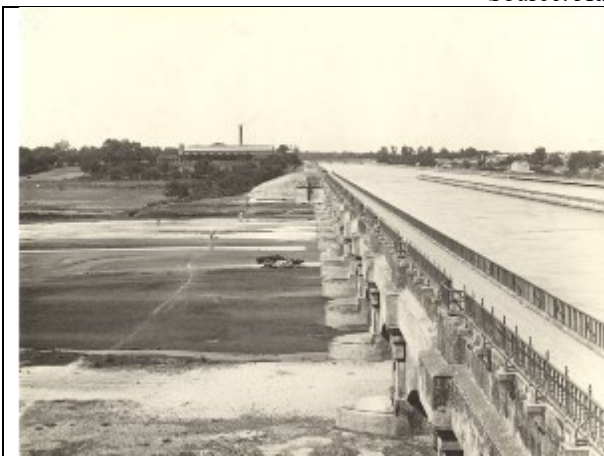
Fig. 42: Archival photo of the Solani Aqueduct, Roorkee.
