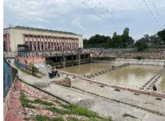
Fig. 24: Pathri power house.
