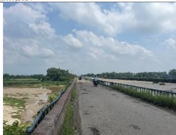
Fig. 43: Current view of the Solani aqueduct, Roorkee.
