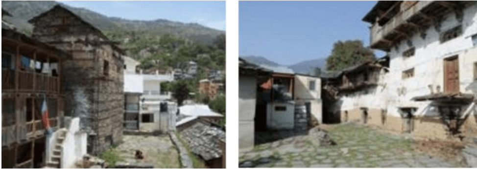
Fig. 9: Traditional Dwellings with Stone & Timber Construction Technique Source: Author, 2012
