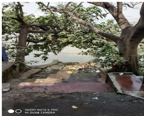
Fig. 14: The Ghat is dumped with wastages.
