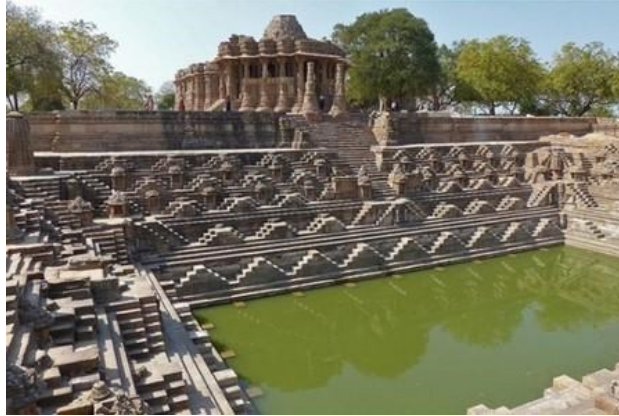
Fig. 8: Use of an exemplary water conservation technique at Kund of part of Sun Temple
