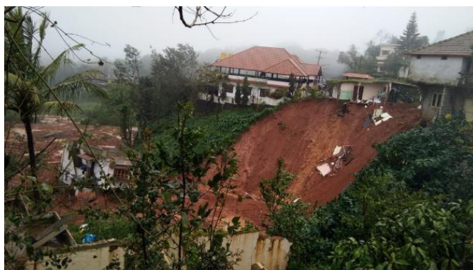
Fig 9: Landslide in Kodagu in 2018,
