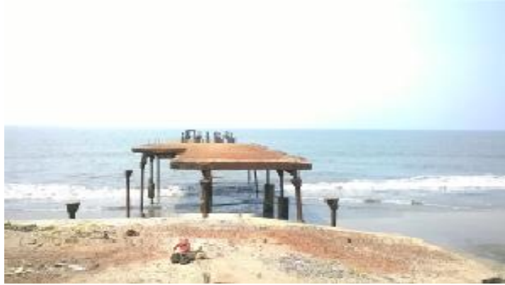
Fig. 8: Old South Pier in Kuttichira- Present Day Source: Author 1
