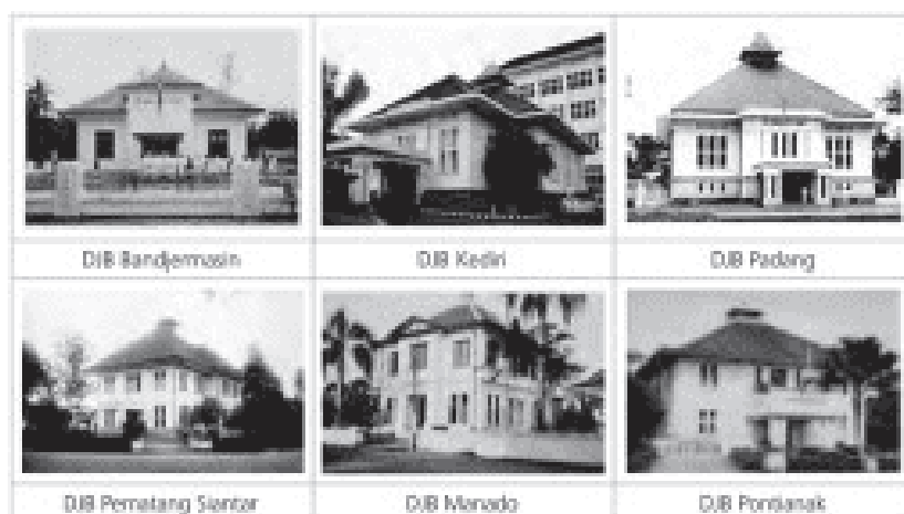
Fig. 9: De Java Bank Building in Indonesia
