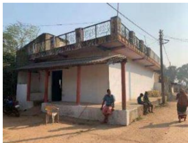
Fig. 13: Addition of a new structure
