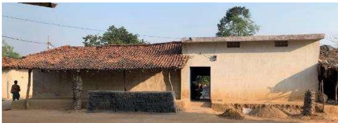
Fig. 14: Completely transformed structures
