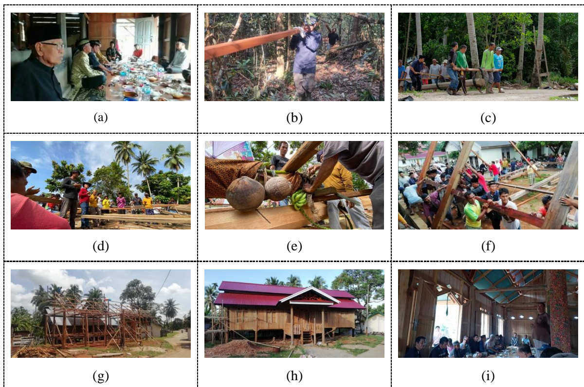
Fig. 5: Godang House Construction Process in Koto Sentajo: (a) Traditional Meetings attended by customary Leaders, (b) Collecting Wood from the Forest, (c) Processing Wood into Poles and Preparation for Establishment, (d) Prayer before Erecting, (e) Symbols on Tiang Tuo (old poles), (f) Enforcing Tiang Tuo and others Poles, (g) Building the Godang House, (h) Completion of the Construction of the Godang House, (i) Raising the Godang House (Thanksgiving for Slaughtering the Buffalo/Cow)
