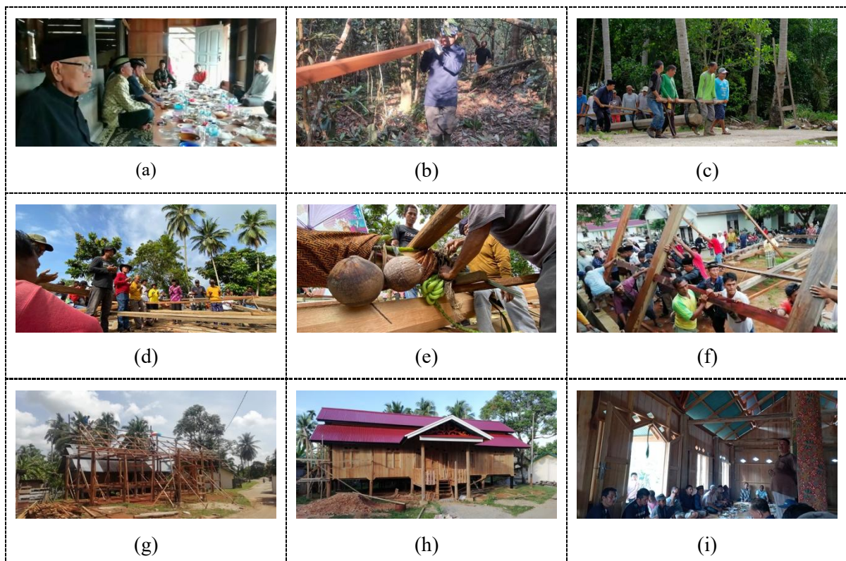
Fig. 5: Godang House Construction Process in Koto Sentajo: (a) Traditional Meetings attended by customary Leaders, (b) Collecting Wood from the Forest, (c) Processing Wood into Poles and Preparation for Establishment, (d) Prayer before Erecting, (e) Symbols on Tiang Tuo (old poles), (f) Enforcing Tiang Tuo and others Poles, (g) Building the Godang House, (h) Completion of the Construction of the Godang House, (i) Raising the Godang House (Thanksgiving for Slaughtering the Buffalo/Cow)
