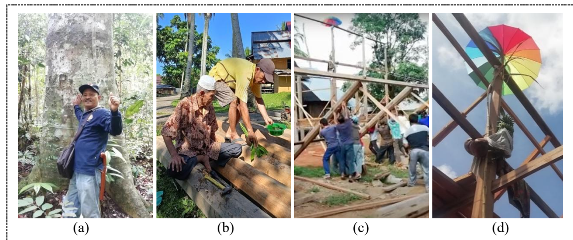
Fig. 7: (a) Timber Felling, (b) Cocak Paek/Tepung Tawar (Spells/Prayers), (c) The Erection of Poles, and (d) Giving Ornaments to Old Poles ( Tiang Tuo )
