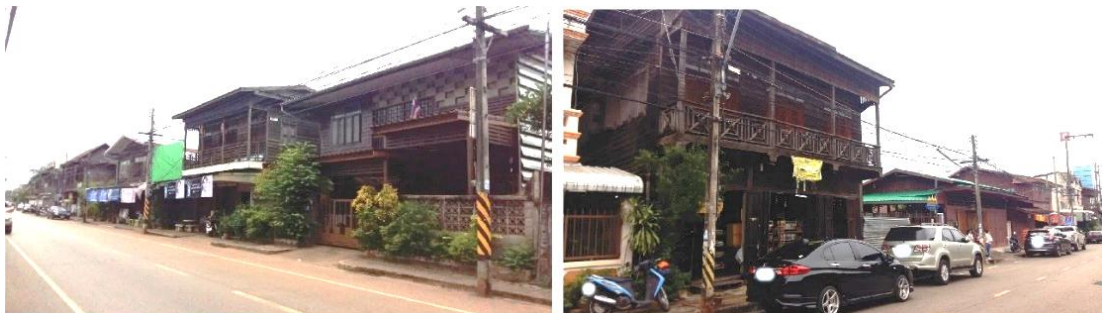
Fig. 8: Vernacular row houses distributed along the main road
