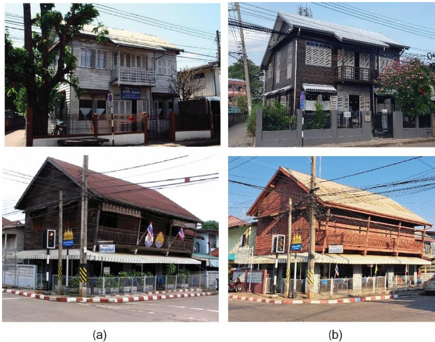
Fig. 9: (a) vernacular row houses before renovation in 2007 and (b) the vernacular row houses after renovation by building owners in 2022.
