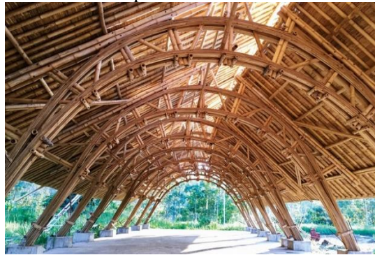
Fig. 7: Trusses/ roof Source: Yadav, 2021
