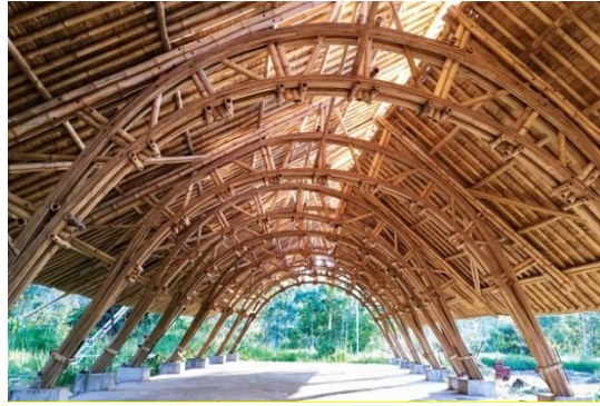
Fig. 7: Trusses/ roof Source: Yadav, 2021
