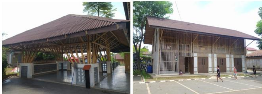
Fig. 11: Bale Alit and Bale RW Building Source: Author, 2022
