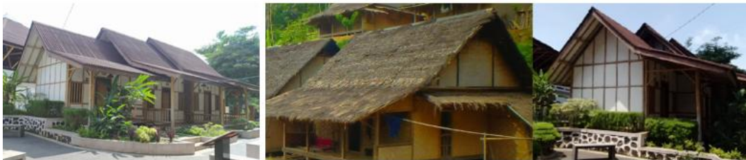
Fig. 9: Building exterior and roof of Bale Motekar Source: Author, 2022
