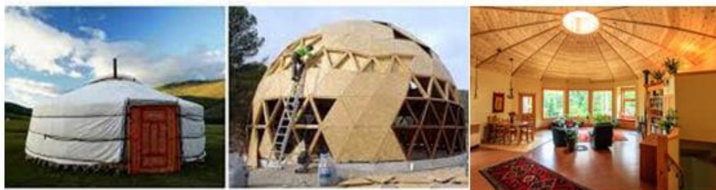
Fig. 1: From the Mongolian yurt to the domed house and its interior Source: Mobile architecture..., 2009.
