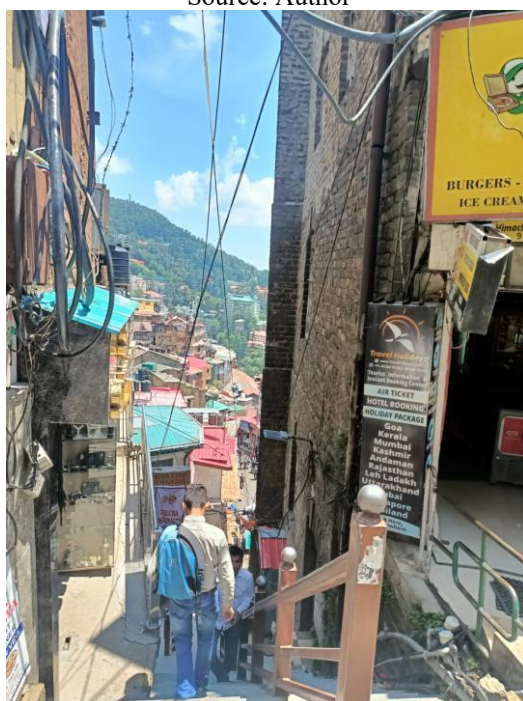
Fig. 18: Steps leading from the mall road to the lower bazaar - view demonstrating the extent of built up congestion
