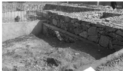
Fig.15: Stone Foundation Source-Author
