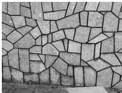
Fig.14: Stone Foundation Source-Author
