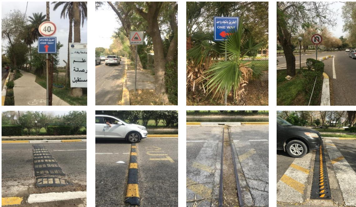
Fig. 6: Poor visibility of traffic signs and speed reduction humps.
