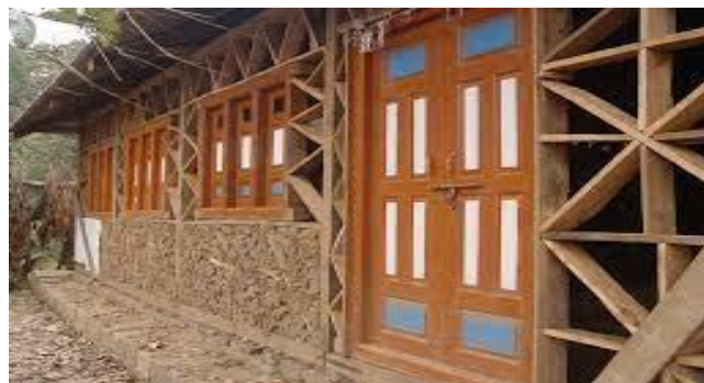
Fig. 4: Dhajji Diwari Construction in Himalayan Region of Kashmir Source: UN habitat and SDC.
