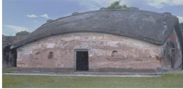
Fig. 2: Chala roof in rigid material at Fatah Khan Tomb, Gaur, Malda, West Bengal, India. Source: Naveen Nishant, 2023
