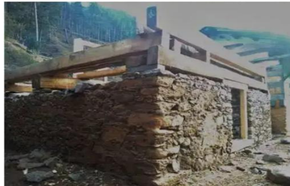
Fig. 3: Koti Banal Construction process (Uttarakhand) Source: Saraswat, 2017.
