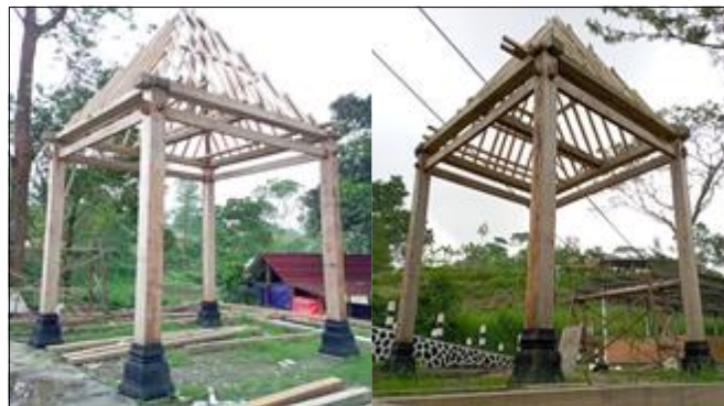
Fig 1: Structure System of a Joglo Traditional Building.
