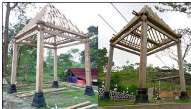
Fig 1: Structure System of a Joglo Traditional Building.
