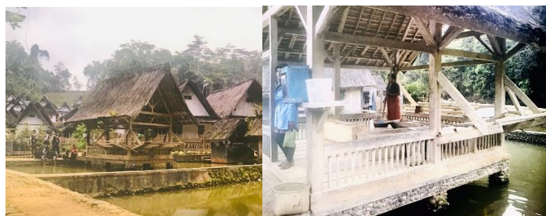
Fig. 13. Saung Lisung in Kampung Naga Source: Sudarwani et.al, 2022
