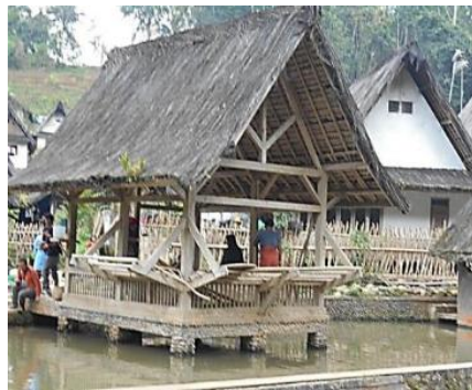
Fig. 4: Saung Lisung in Kampung Naga Source: Sudarwani et.al, 2022
