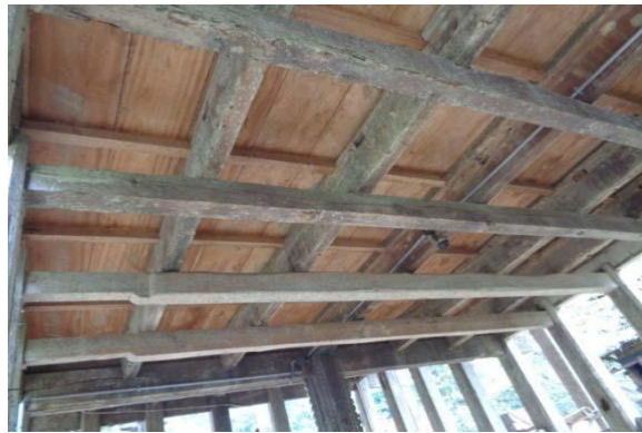
Fig. 10: Tongkonan beam construction
