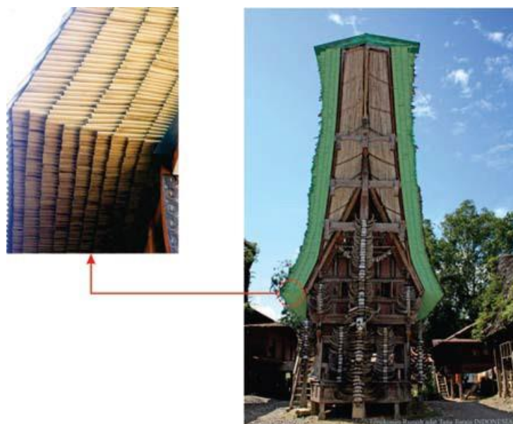
Fig. 7: Visual construction form in roof envelope
