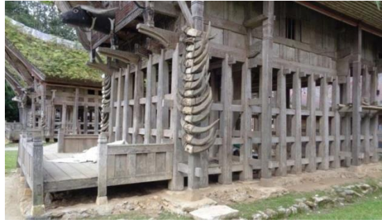
Fig. 8: Tongkonan pile construction
