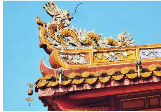
Fig. 13: sword heads at roof angles on Five-Phoenix Pavilion roof Source: Xuan Dat, 2022
