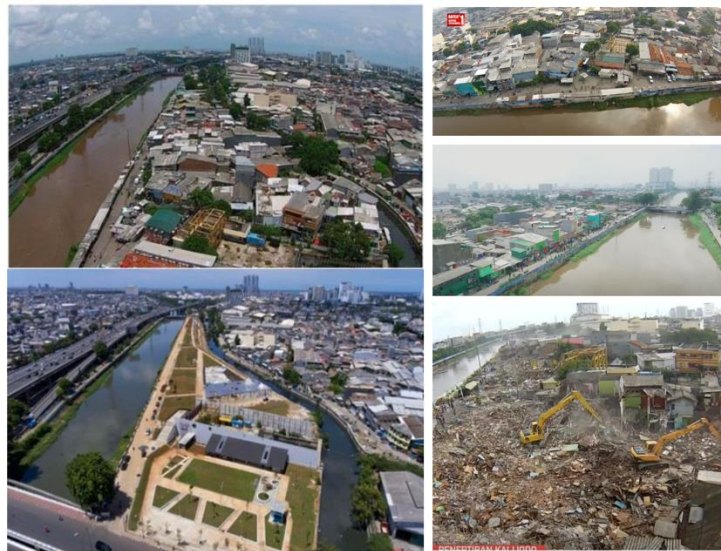
Fig. 7: Transformation of the illegal settlement becoming a public space Source: Authors
