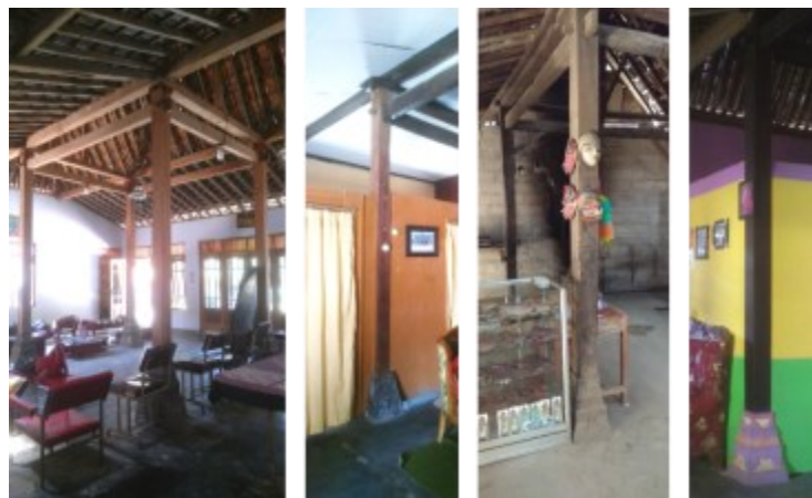
Fig. 6: Saka guru in some houses Source: Author, 2021
