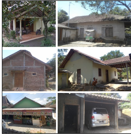
Fig. 8: Some new buildings Source: Author, 2021
