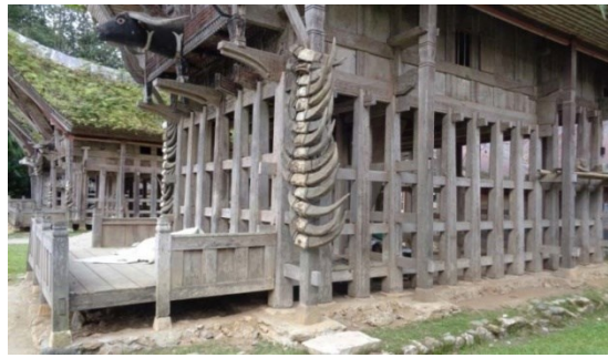
Fig. 8: Tongkonan pile construction Source: author
