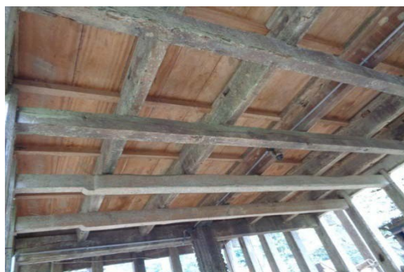
Fig. 10: Tongkonan beam construction Source: Author
