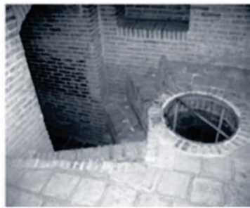
Fig. 5: Underground communication passages of linking underground space with the spaces of the house Source: Lavafpour, 2015
