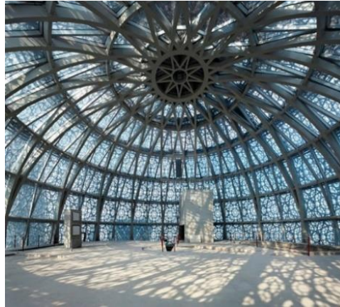
Fig. 11: Dome completion of the openwork clothes of the tower
