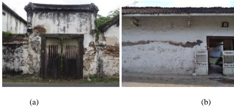
Fig. 3: (a) Facade Conditions in Small Gate House buildings, (b) Facade Conditions in Large Gate House buildings. Source: Author
