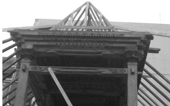
Fig. 5. The roof rested on a series of beams ( blander and pengeret ) placed at the ends of saka (pillars)
