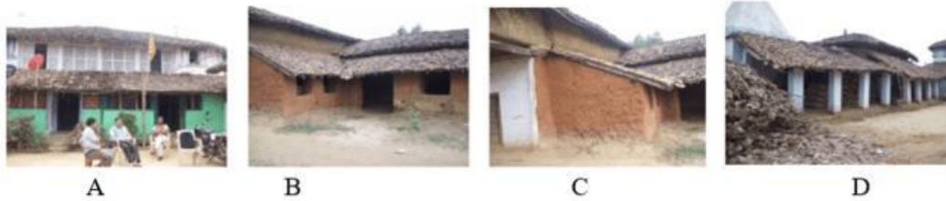
Fig. 12: House 1(A) Double storey structure (B) Stable & store (C) Fodder store in front & farm equipment store at back of house (D) Store with a corridor and columns in brick & mud mortar.
