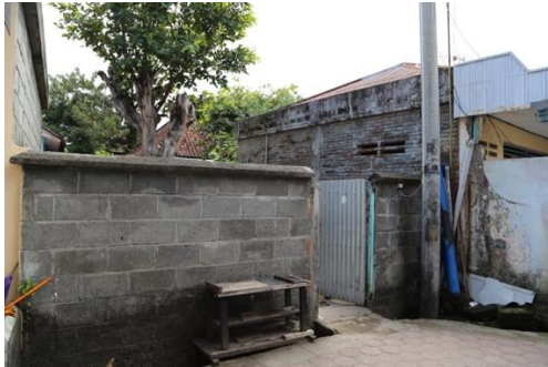
Fig. 2: Main entrance gate Source: Authors, 2018
