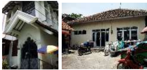
Fig. 7: At Taqwa Mosque and the RW hall in Kampung Kulitan Source: Author, 2022
