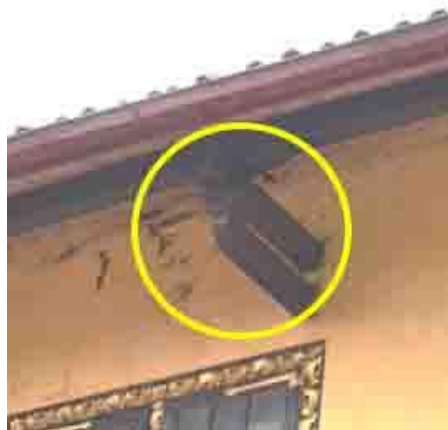
Fig. 18: Fukien type on the Roof Trellis on the Second Floor of Keraton Sumenep's Main Building Source: Author
