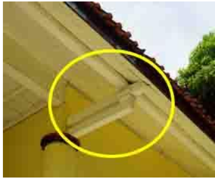
Fig. 19: Fukien type on the Roof Trellis of Heirloom Storage Building Source: Author
