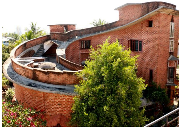
Fig. 6: Typical example of Laurie Baker's architecture – Centre for development studies, India (Source: Deccan Herald)
