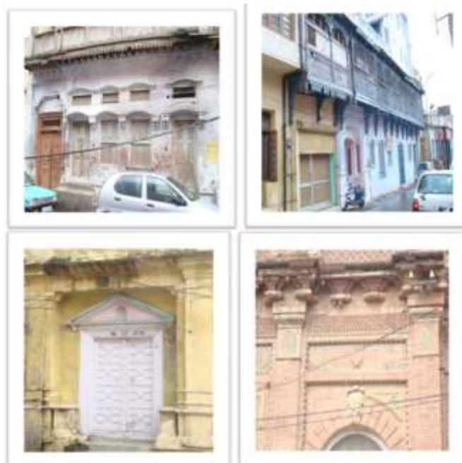
Fig. 5: Visual survey of old Jammu city - traditional dwellings
