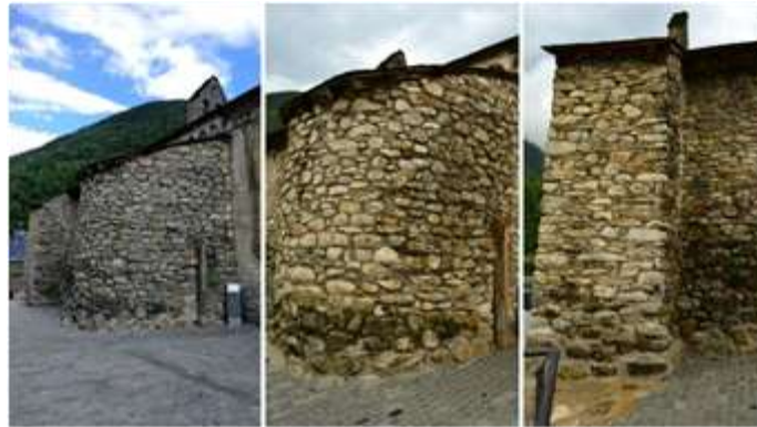
Fig. 15. Passive thrusts of the buttressing elements.
