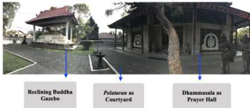
Fig. 2: Image of the Prayer Hall and Pelataran at Vihara Mendut Source: Author
