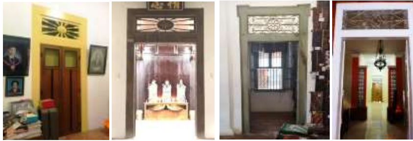
Fig. 5: Various Ventilations of Lasem Door
