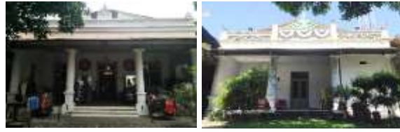
Fig. 7: Type of Lasem house with neoclassical columns and gable/gabletoppen Source: M. Maria Sudarwani, Edi Purwanto, R. Siti Rukhayah
